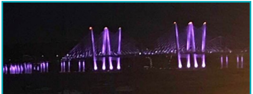
The Governor Mario M. Cuomo Bridge was lit up in purple in recognition of Domestic Violence Awareness Month.
